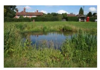
Farley Green Pond in Albury is the last of seven balancing ponds that take water from the local roads. It plays a vital role in helping to avoid the flooding of nearby homes, but its effectiveness has been hampered by the sand and soil that flow in with the water and cause it to silt up.
